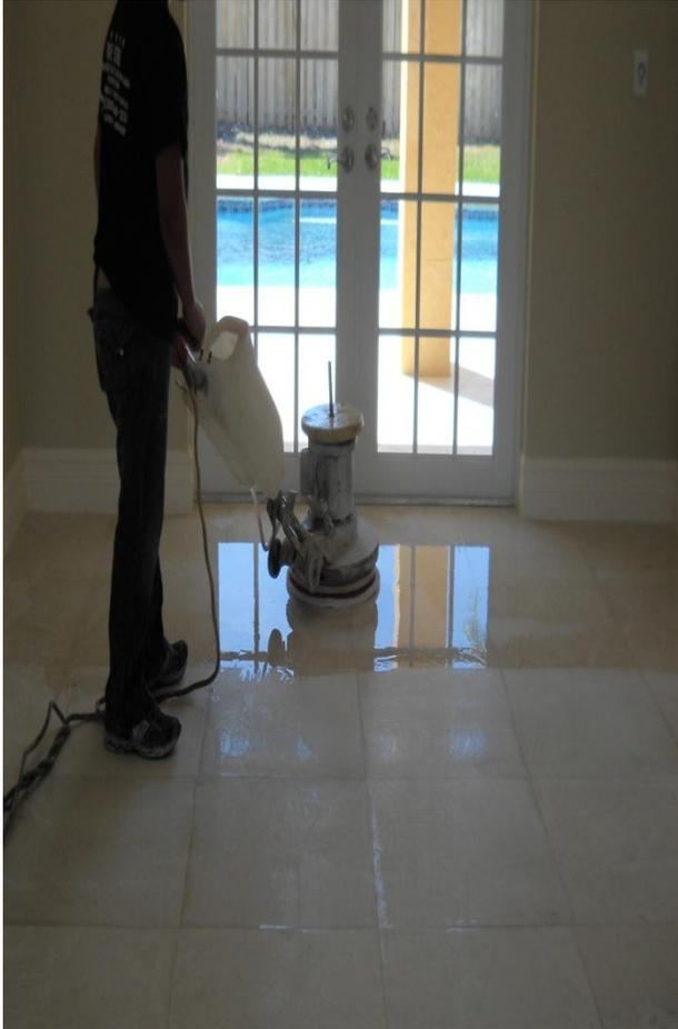
Simply put, the crystallization process works by forcing one ion from one molecule to another in the cement matrix that holds the crystals together. This forms a new cement matrix that can be harder than the original cement matrix of the stone. The newly hard and the preexisting softer structures form two layers, and thus a layer of separation is between them.
