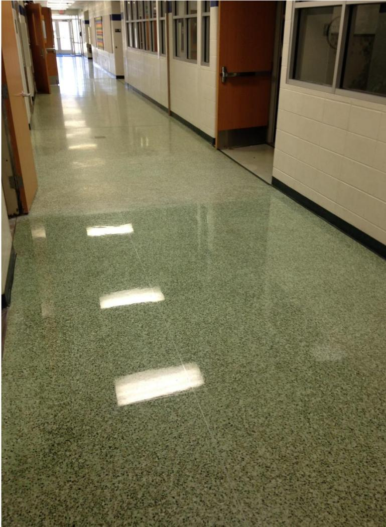
Obviously, one would not want to use crystallization on a honed, non-reflective surface. This process is meant only for polished surfaces. If one is confronted with maintaining a large polished marble or terrazzo floor with high foot traffic, an excellent way for maintaining this polish, more times than not, will be crystallization.
